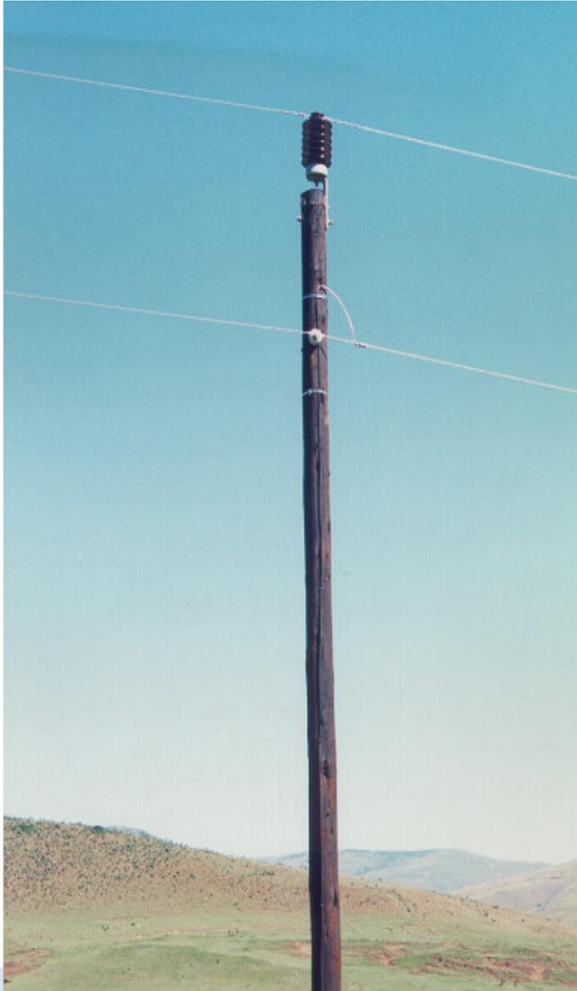
Intermediate structure with under strung earth wire.
